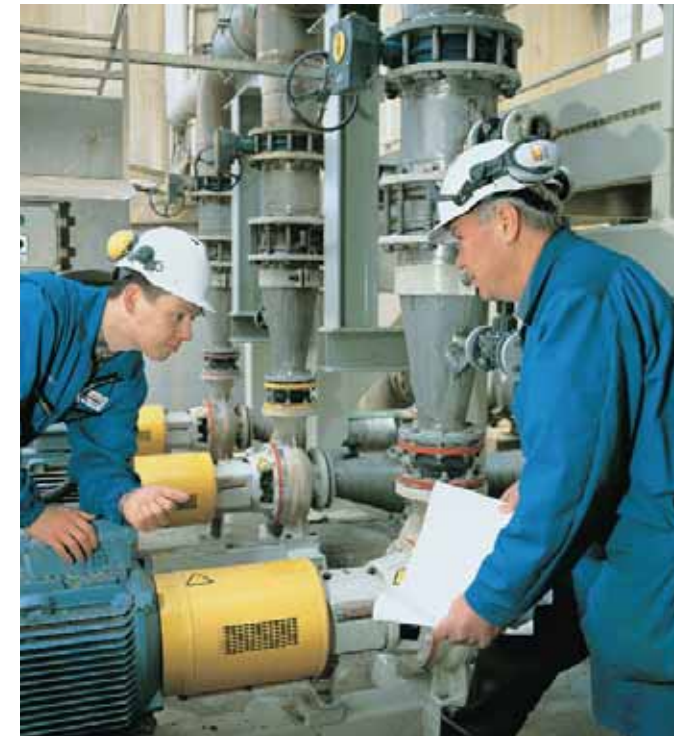
Following an energy audit at one of its pumping stations, West of Scotland Water expects to make savings in electricity costs of £80,000
