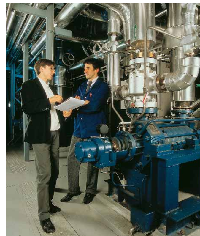
During an initial meeting the audit engineer takes a look at the inventory of motors contained within a plant.
